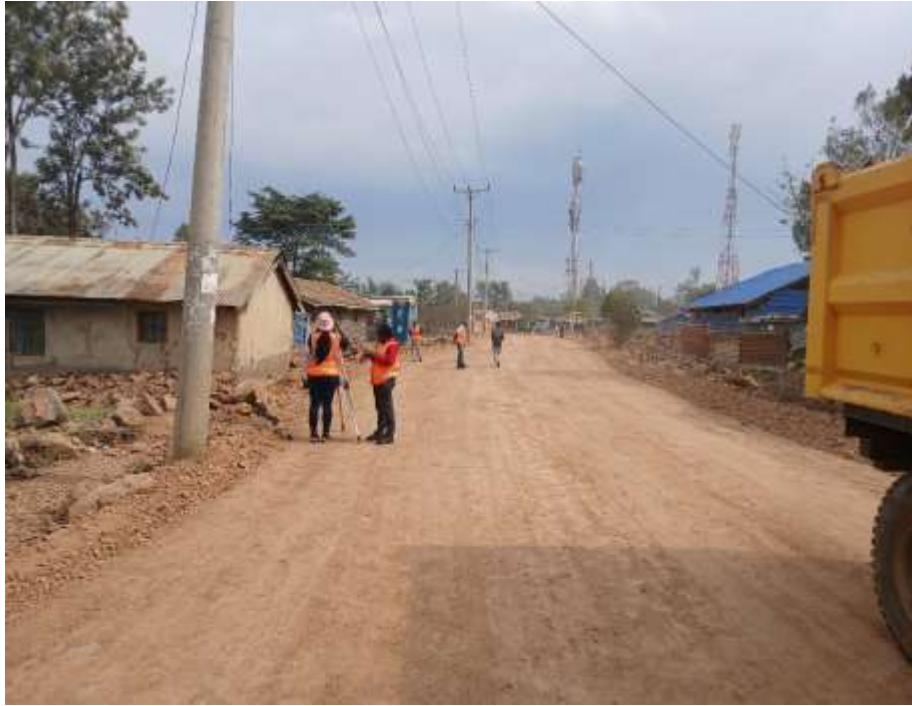
Level check for Subgrade 1 Kaombe-Kasawino Road
