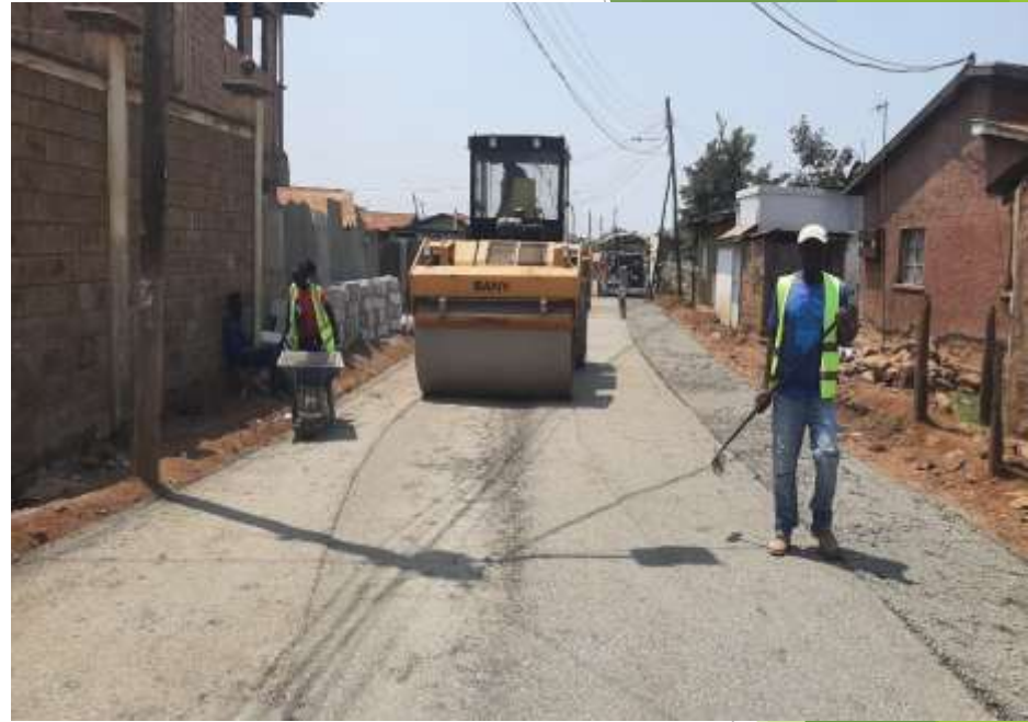
During compaction of GCS Base layer
