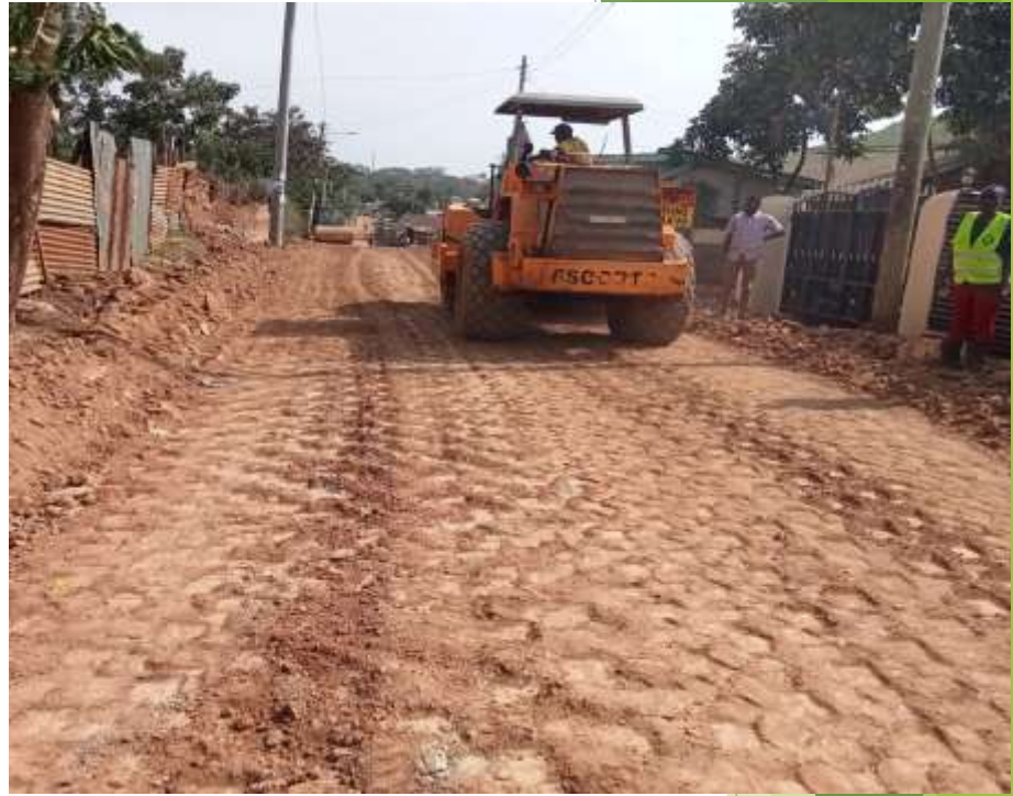
Compaction of subgrade 1 Km 0+260-0+360
