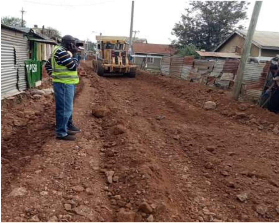
Processing of Subgrade 1 Km 0+660-0+800
