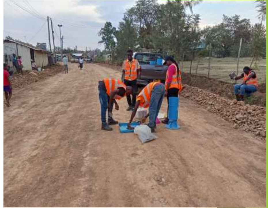
Field density test for subgrade 1
