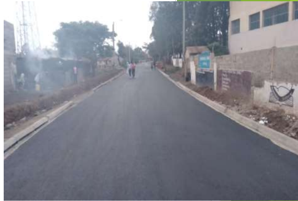
During laying of asphalt
