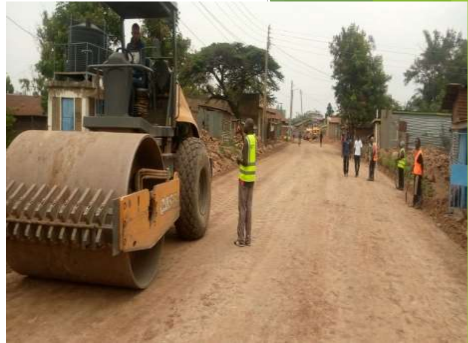
Compaction of subgrade 2 layer
