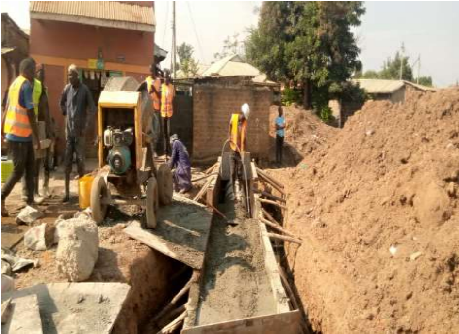
Casting of surround for cross culvert at Km 0+290
