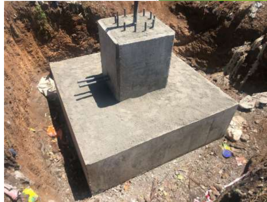
Pad footing and column base casted for the floodlight
