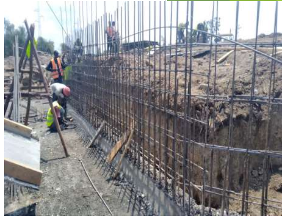
Steel fixing for walls and wing walls for the box culvert
