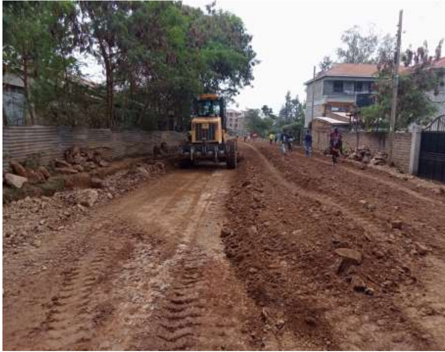
Processing of subgrade 1 Km 0+700-0+800
