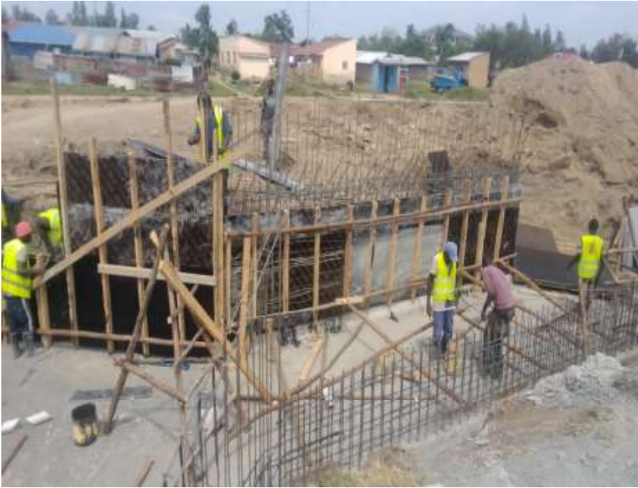
Installation of formwork for Culvert wall
