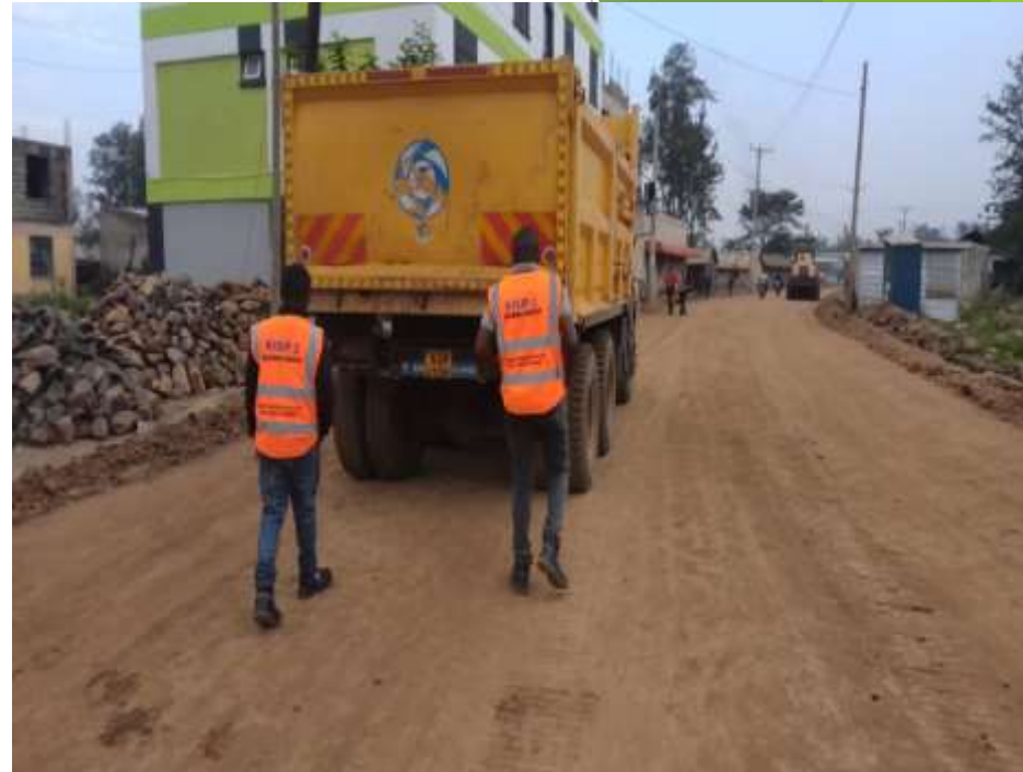
Proof rolling for subgrade 1 (section passed)
