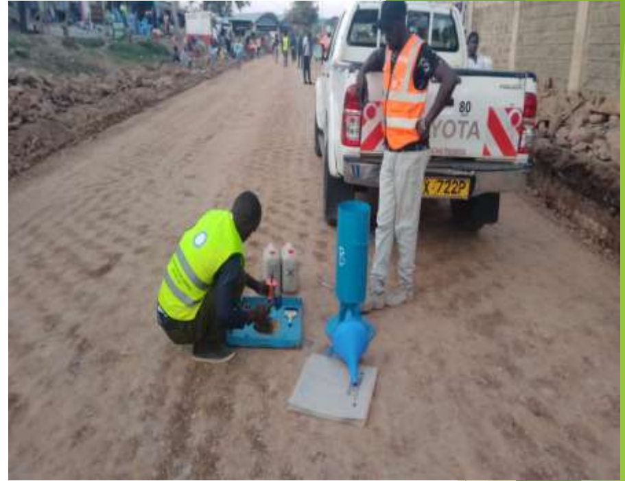
Field Density Test for formation layer Highway Sec School-Mama Ngina Road
