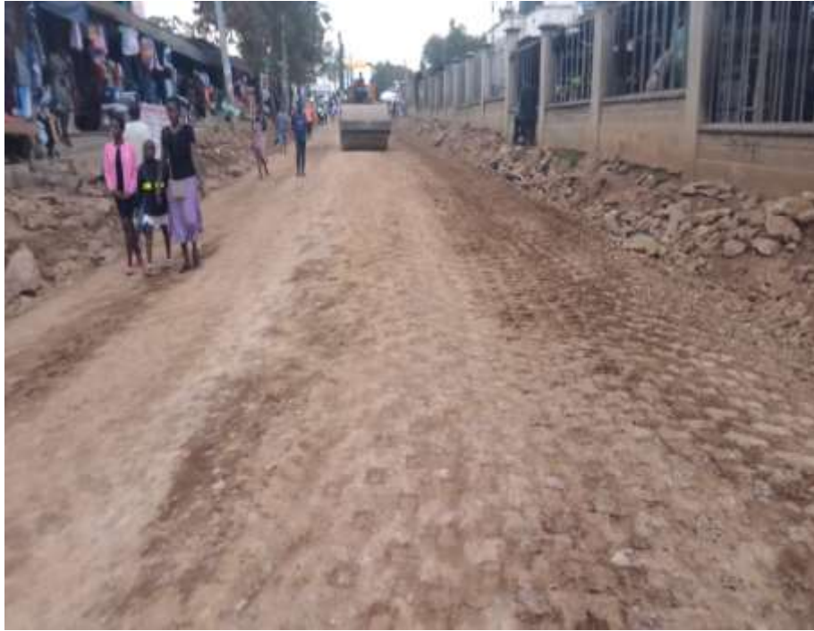
Compaction of subgrade 1 at Highway Sec-Mama Ngina Road
