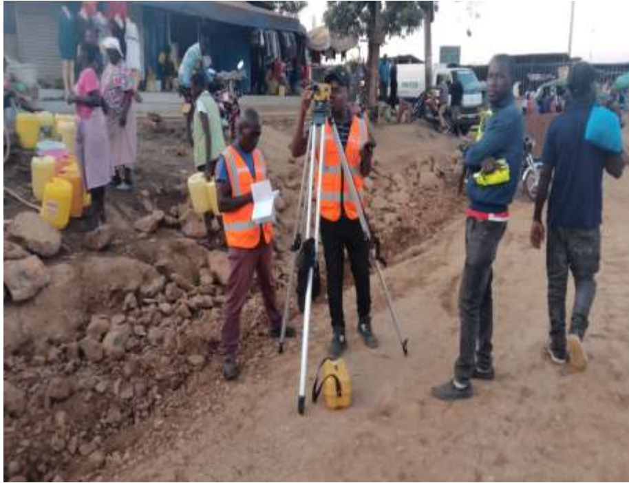
Level check for formation layer Highway Sec School -Mama Ngina Road
