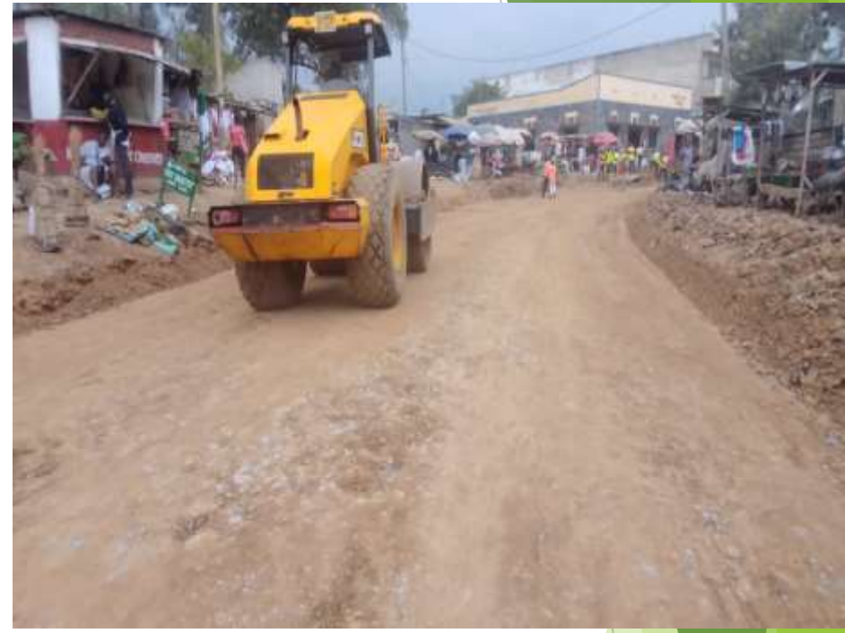
Compaction of formation layer SDA-Thep thep Road Km 0+090-0+200
